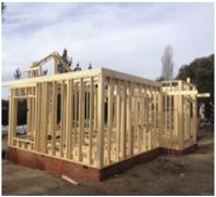
Fig. 1. Timber frame structure
