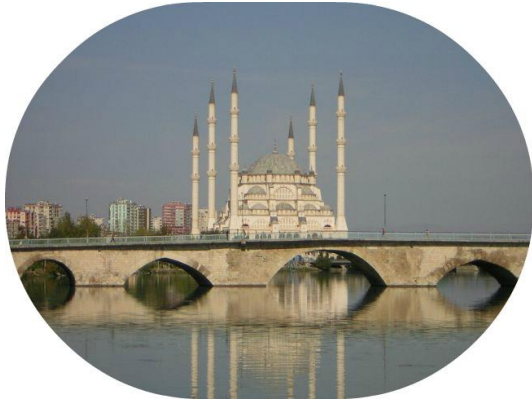
a 4th-century Roman bridge
