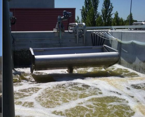
$25 \text{ m}^3$  activated sludge ( $3.5 \text{ g TSS/L}$ ) +  $1.4 \text{ m}^3$  of anammox enriched sludge ( $10 \text{ g VSS/L}$ )
