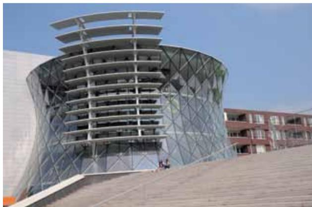
Through its participation in CONCERTO, the Dutch city of Heerlen uses heat energy stored in old mineshafts for the heating and cooling of buildings. The last miner left the mines in Heerlen in 1976. Since then, the former mineshafts have been filled with geothermally heated ground water, which has different temperatures at different depths and can therefore be used for both heating and cooling.
