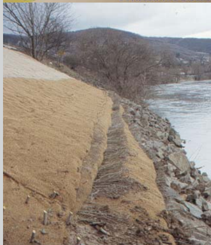
Figure 19: Infill of gravel material into the riprap to avoid loss of soil material and to improve moisture capacity of the underground Figure 20: Geo-textiles covering rip rap
