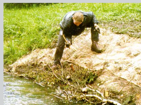
Figure 25 (right): jute mesh is rolled out to protect the just brought out sod from erosion, a dead fascines protects the toe, the jute mesh is fixed with willow stakes
