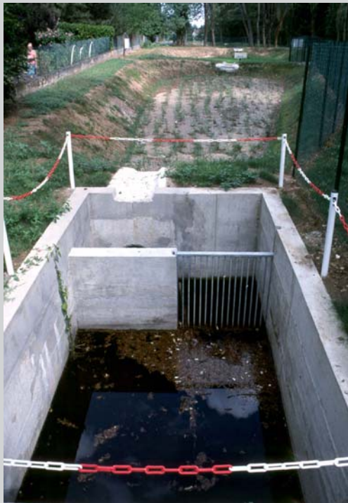
Figure 34: Sand and grit separator of with overfall into the first of three detention and infiltration basins
