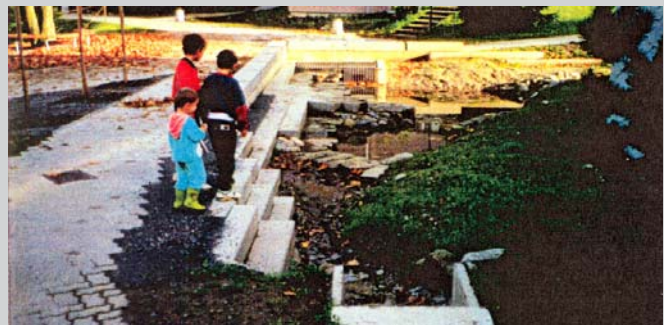
Figure 4: Sections of detention basin at the Sägertenbach, Brook Concept Zurich
