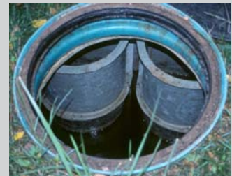
Figure 3a,b (bottom): An intermediate filter system is installed between the third detention basin and the discharge pipe connecting the system with the stream
