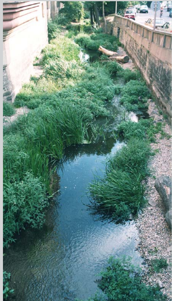
Figure 8: 2003 - The new stream channel instead of old mill race based on geomorphologic modelling
