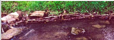
Figure 13: Sketch of a dead fascine, used along the Kaitzbach Figure 14: Dead fascine at the Kaitzbach, about eighth weeks after construction, 1999
