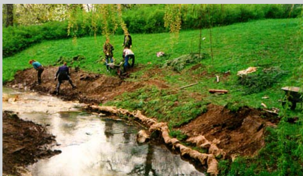
Figure 24 (left): Re-using of sod, jute mesh is still rolled in at the toe of banks
