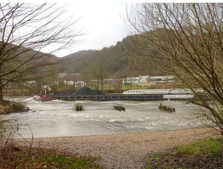
Groynes protect the backwater. Flattened banks offer people opportunities to experience the river (©Municipality of Stuttgart).
