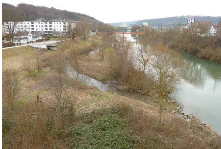
The forelands of the Neckar River were flattened, the woody plants thinned out, a river branch constructed. The housing area Brückenwasen (left) offers residents a high quality of life. (©Municipality of Stuttgart)
