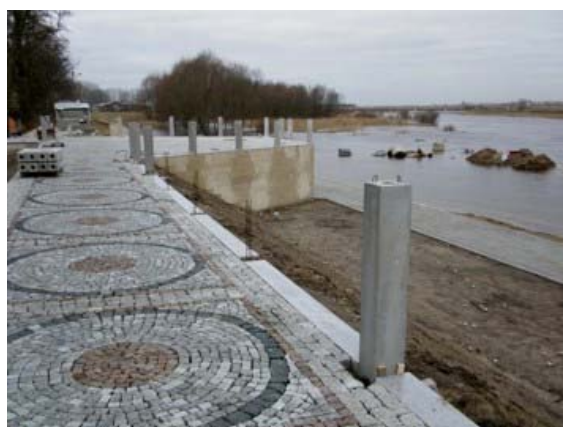
The construction site in August 2010 – paving detail (©J. Kończak)
