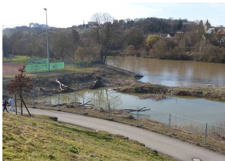
The standing backwater joins the Neckar by a small access. After completion of the second section of construction the water will be able to pass through. (©Municipality of Stuttgart)
