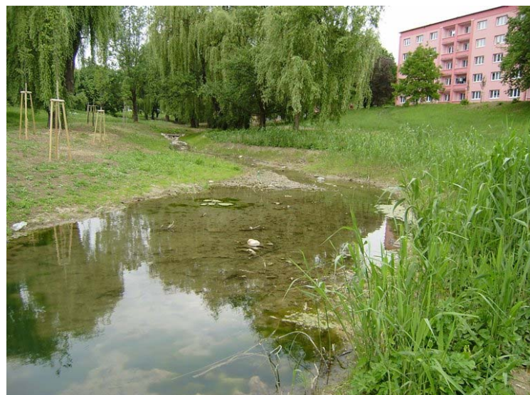
After revitalisation 2009 (©Municipality of Uherský Brod)
