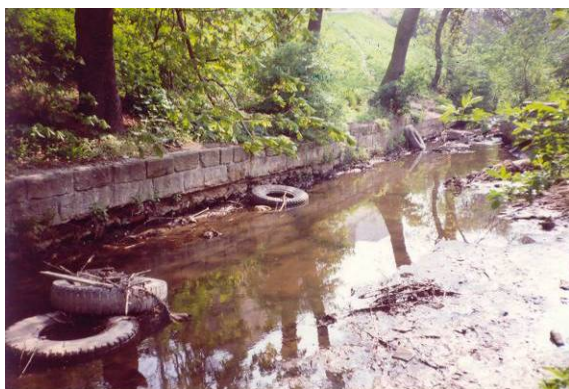
Situation before the revitalisation (©Šindlar, s.r.o.)
