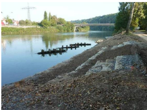
Breakwater structures (fascines made from willow branches) stabilise the banks and support the formation of new structures. Steps facilitate access to the water (©Municipality of Stuttgart).
