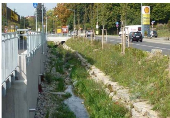
Land was acquired by property exchanges with the neighbouring company (©Municipality of Stuttgart)
