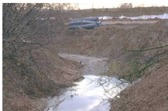
Only a ditch and some initial meanders were built; otherwise the stream was allowed to create its own bed. (©BHM Planungsgesellschaft mbH)
