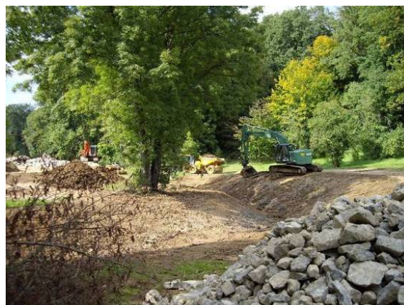
Potentially endangered zones have to be secured with stones. (©Municipality of Stuttgart)
