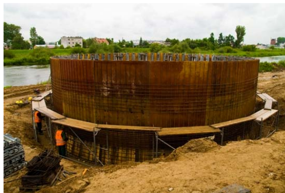
Work on the project implementation in 2010
