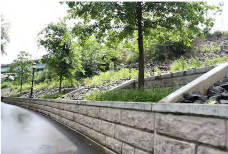
Figure 15. Mortensen Riverfront Trail. Trees planted along the riverfront’s dike needed to be encased in concrete to prevent their roots from compromising the earthen structure.
