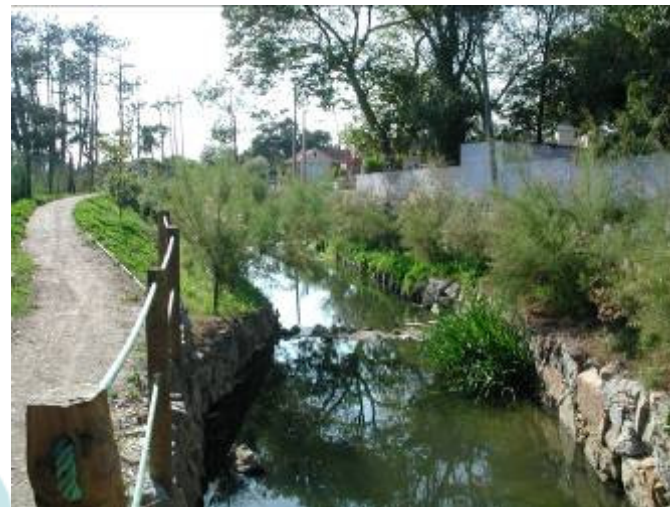
Rehabilitation of urban creeks, Gaia, Portugal
