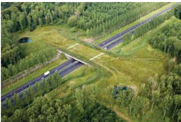
Figure 4.2 Two examples of overpasses in combination with fences across a four-lane motorway (left) and a motorway under construction (right) from the Netherlands
