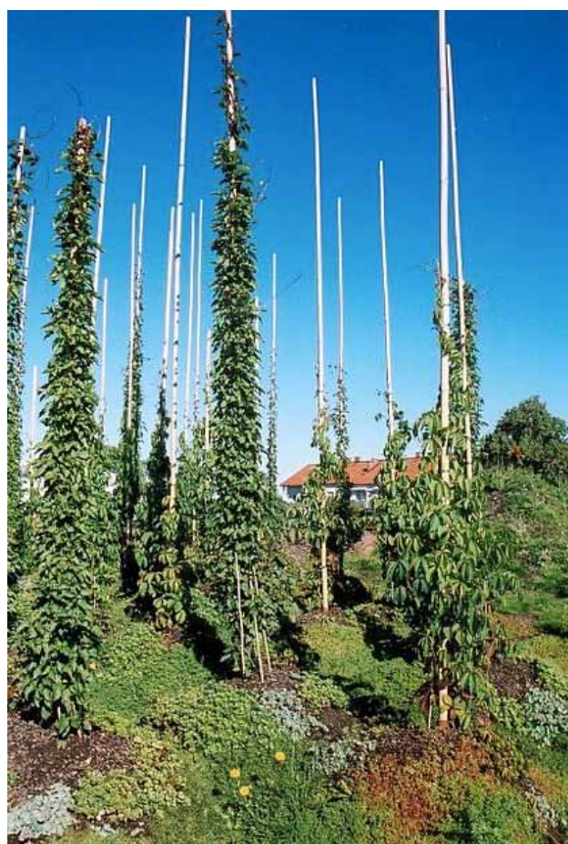
All new, and some existing buildings in the neighbourhood, have green roofs, including the largest green roof (9 500 m 2 ) in Scandinavia. They create valuable habitats and intercept half of the total rainfall. (Photo: Scandinavian Green Roof Institute)
