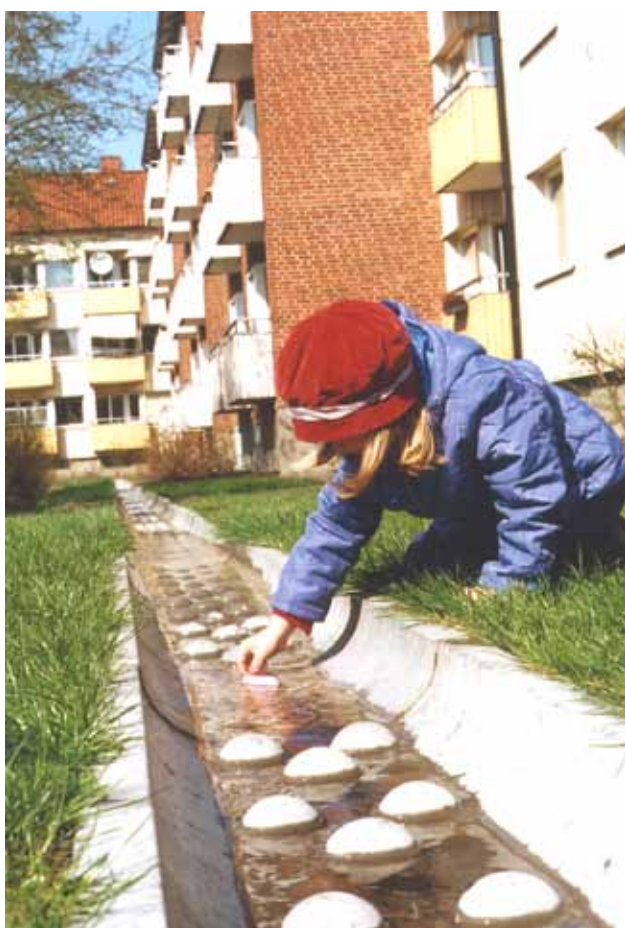
In the new storm water system, 70 % of all rainwater from rooftops and other impervious surfaces is collected from gutters and channelled through canals, ditches, ponds and wetlands before finally draining into a traditional closed subsurface storm water system. (Photo: John Dolocek, City of Malmö)
